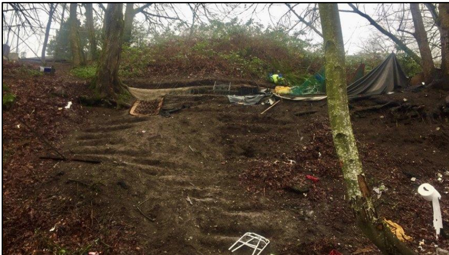
Photos 6 and 7. One steep slope before and after encampment vacation and ecological restoration at the project site. Erosion control blanket and native trees, shrubs, and ground covers were installed to improve stormwater and habitat benefits over time.
